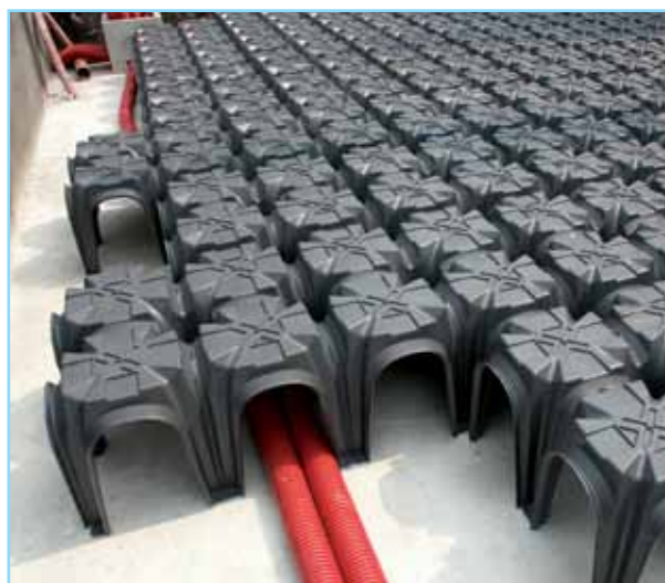
fig. 4) Installation of the MODULO FREEZE
