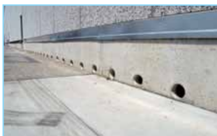
fig. 5) Appropriate external ventilation - Holes approx. every 1 m.
